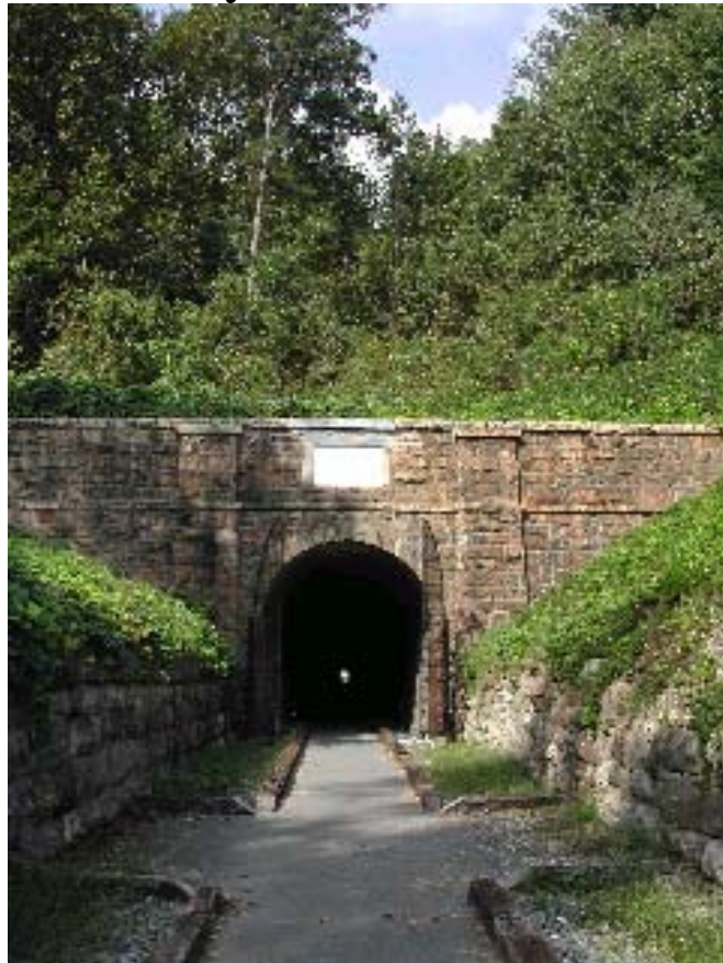
Western and Atlantic Railroad Tunnel
