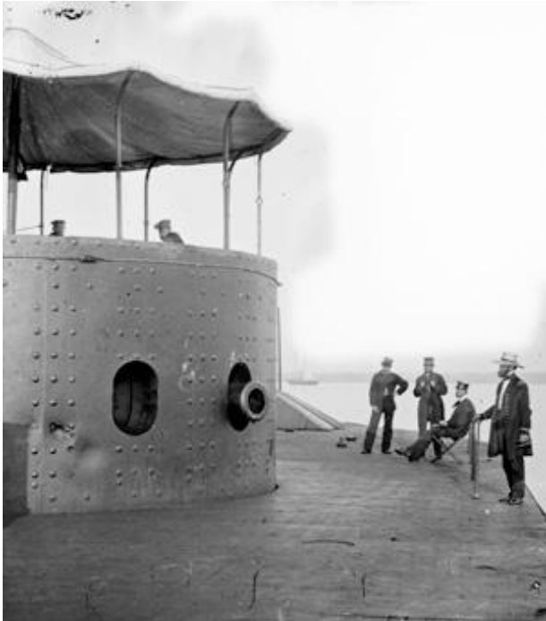
Close up of the USS Monitor's turret (Library of Congress)
